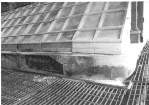
图 3 电解槽侧角部槽盖板外观 Fig.3 The appearance of the side angle of the electrolytic cell
